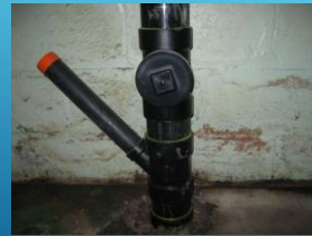
Stack Cleanout's no longer required
